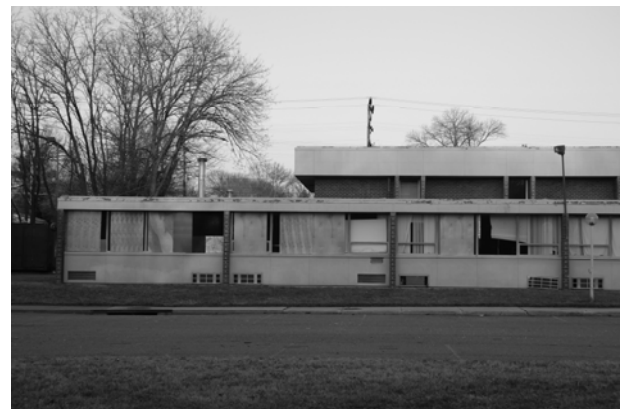
Recent photo showing boarded up windows at MCAD.
